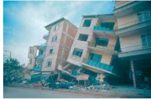
Sway mechanisms are often inevitable with soft storey ground floors (Izmit, Turkey 1999).
