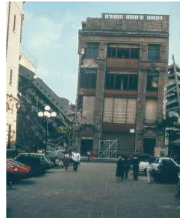
The modern reinforced concrete building to the left collapsed after pounding against the older very stiff building to the right (Mexico 1985).
