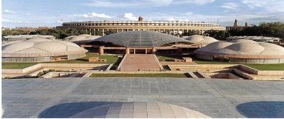
Fig.1 Parliament Library building with FR HPC (50 MPa) bubble type units.
