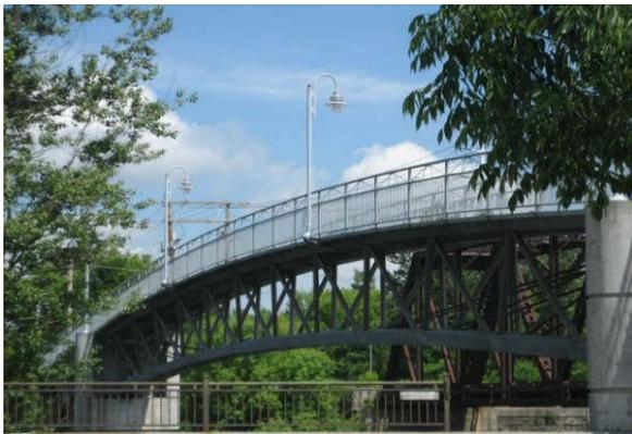
Fig.3 The Sherbrooke Reactive Powder concrete Footbridge, Quebec, Canada.
