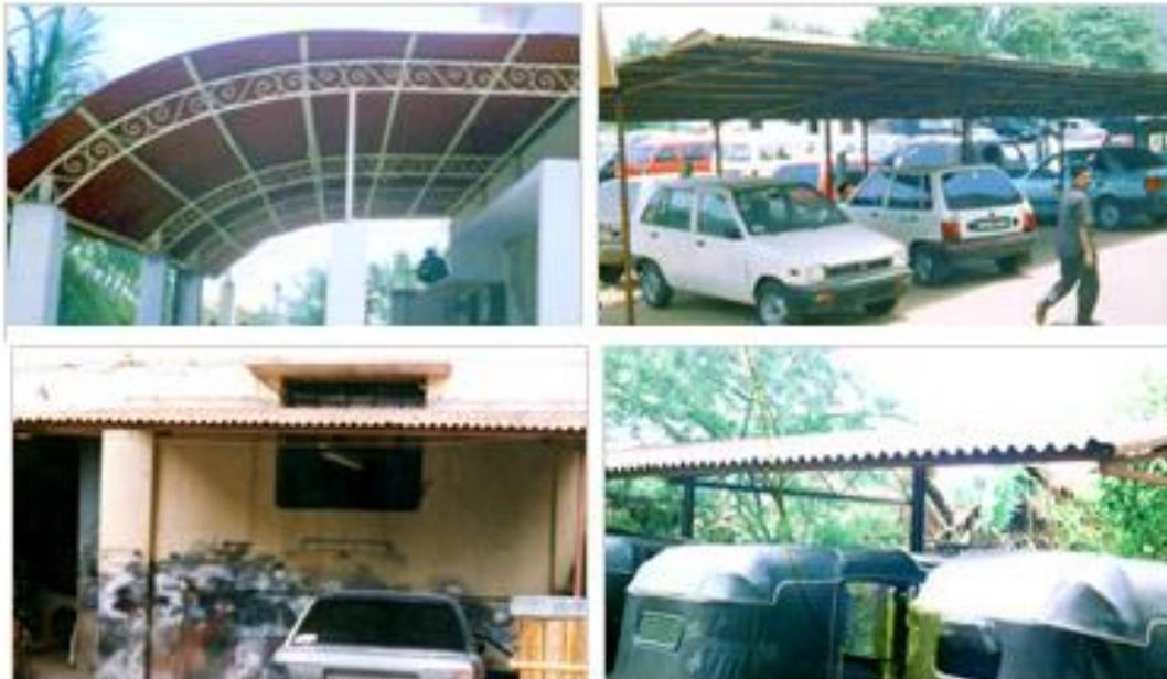
Fig.2 Red mud plastic sheets for roofing
