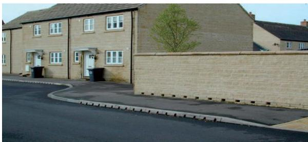
Fig.3 The openings in the property wall and road on the new estate which is in a known area of flood risk, were specifically designed to convey flood flows away from the property and into temporary underground storage.
