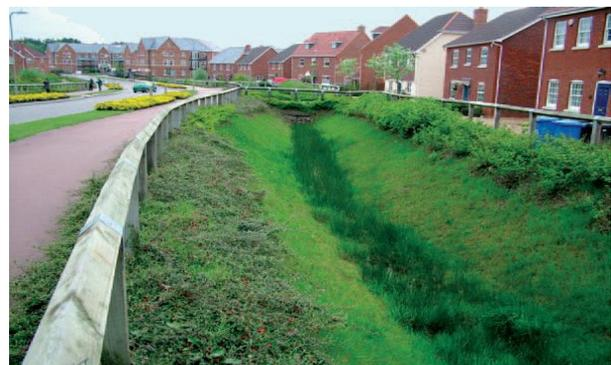
Fig.4 A swale used to deal with surface water drainage in a housing development in England.
